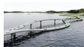
Pearl River Necklace bridge: a twisted solution to an unusual traffic problem
