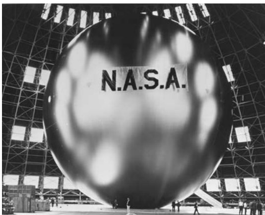
Fig. 8 Echo II rigidizable space inflatable envelope (courtesy of NASA).
